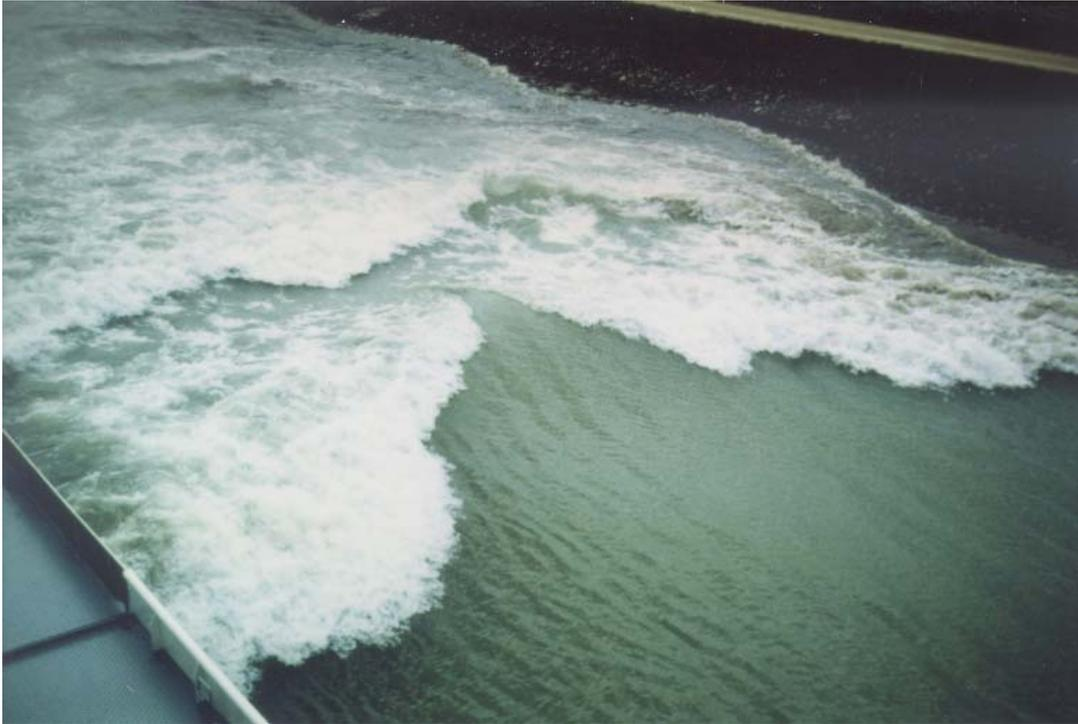
Fig 8 – Wash waves on a canal slope
